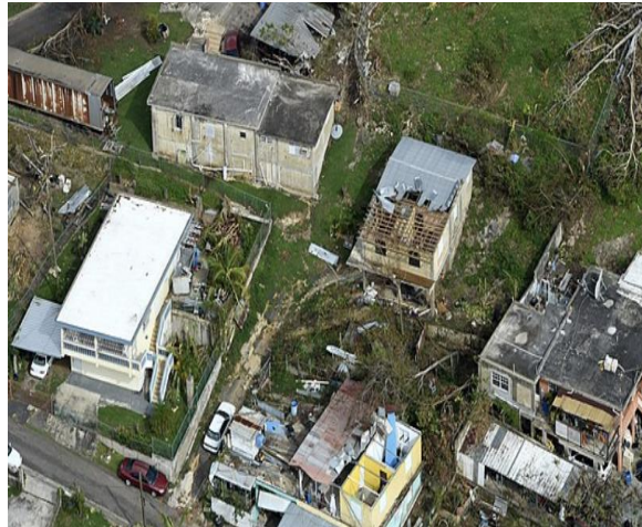
Photo of a damaged area caused by hurricane
